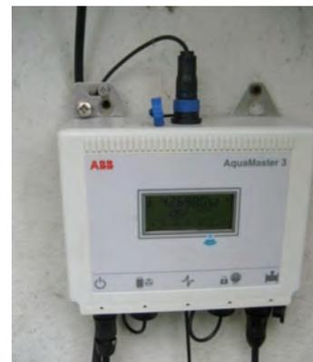
Using solar-powered water meters can have a number of benefits; improving the continuity of measurement for leakage and consumption, and reducing the electric consumption - therefore the carbon footprint which is generated by business activity, an issue close to the heart of many.
