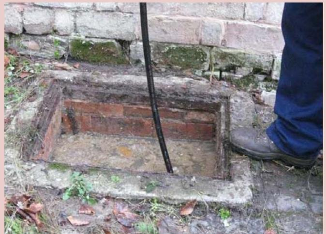
**Water Company staff clearing a blockage on a transferred sewer**
